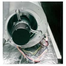
Easy to remove blower housing for quick service and General Electric ECM variable speed motor
